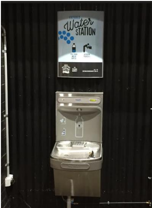
Figure 2: City of Melbourne Hydration Station
